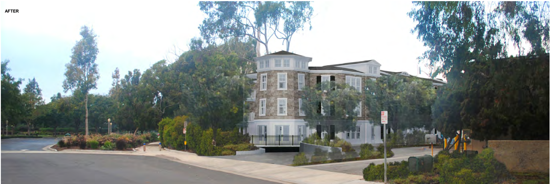
Exhibit 9D: View Location 4 - Looking Northwest Towards Project Site Ford Road Residential Project
